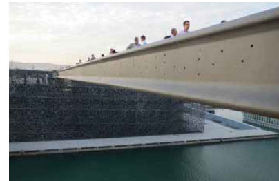
Post-tensioned UHPC channel girder in the MuCEM pedestrian bridge, Marseille, France (photo courtesy of Ben Graybeal)
