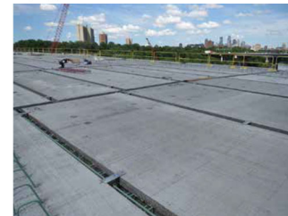
Precast deck panel placement prior to UHPC connection casting, Franklin Avenue Bridge, MN (photo courtesy of Ben Graybeal)
