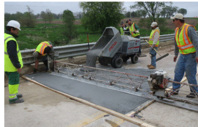
Figure 1. UHPC overlay construction in Buchanan County, Iowa.
