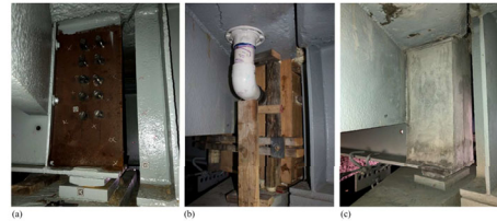
Fig. 16. Use of UHPC for the repair of deteriorated bridge girder ends in Connecticut in 2019: (a) girder end preparation; (b) formwork; and (c) completed repair. (Images by Arash Zaghi.)
