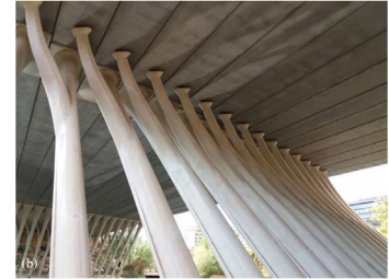
Fig. 8. La République Bridge in Montpellier, France, with (a) overall structure (Image courtesy of Agence Rudy Ricciotti); and (b) slant columns and ITE® beams from below. (Image courtesy of François Toutlemonde.)
