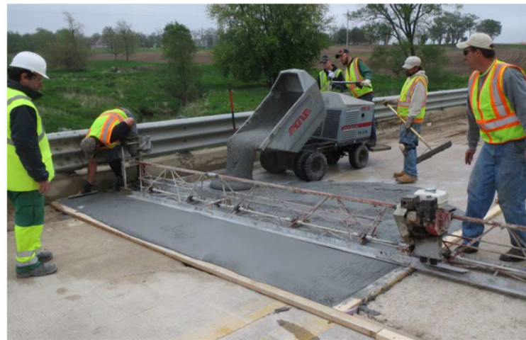
Fig. 14. One of the early implementations of UHPC overlay repair in 2016 in Iowa. (Image by Benjamin Graybeal.)
